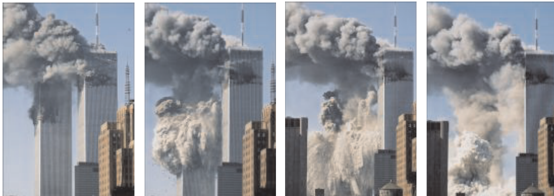
9:59AM THE LEVELING OF WORLD TRADE CENTER SOUTH (WTC-2)
